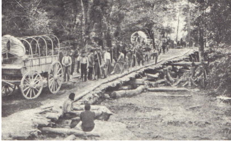
Corduroy Road (You can see a section of one at the White Oak Civil War Museum.)
